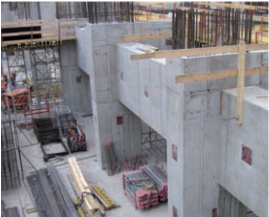
Anchor channels in elevator shaft or stairway
