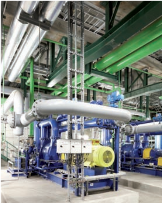
Fastening of heavy machinery
