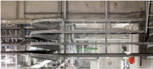
Fastening of cable trays
