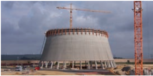
Power plant under construction
